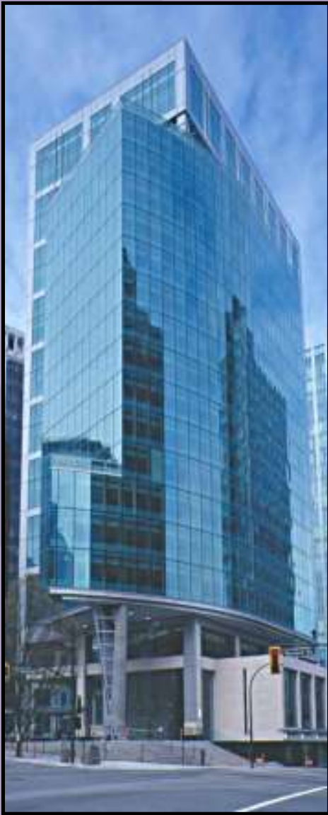
All the glass in this tower at 401 Burrard Street in Vancouver is typical of the product produced by Garibaldi.
