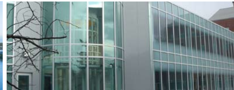
UNIVERSITY OF VERMONT MULTI-SEASONAL DESIGN IMAGE BURLINGTON, VT ARCHITECT: JOHN ANDERSON STUDIOS
